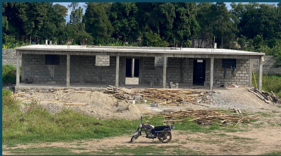
Outdoor Classroom Construction to begin March 2022
